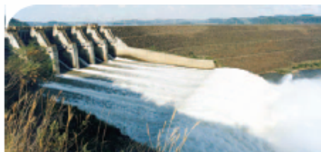
Left to right: Bello Santiago hydroelectric plant - Brazil Rodenhuize thermal plant - Biomass - Belgium Researcher at CIRSEE - France
